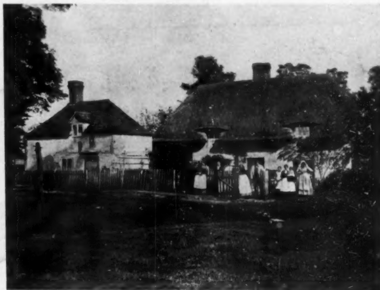
The charm of the English cottage roofs is due to their unbroken surface. Note the difference between the lines of the slate and thatch
