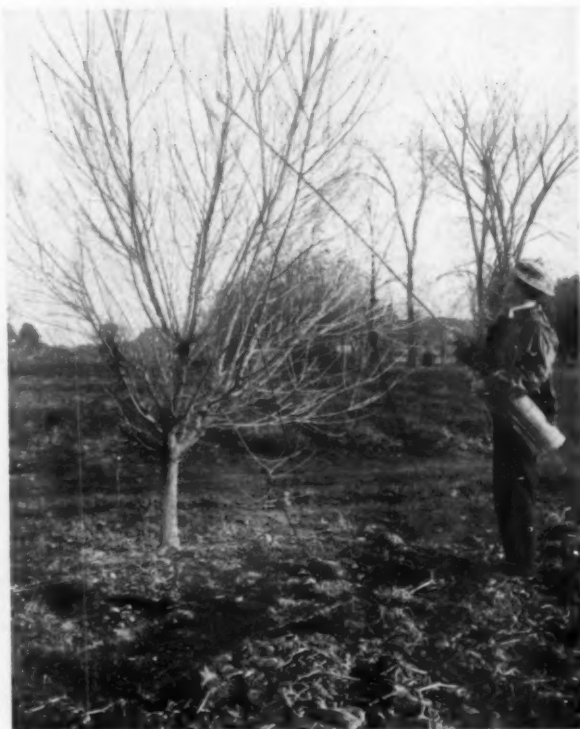
A compressed-air sprayer is a great convenience for applying the liquid insecticides; for the orchard an extension rod may be used to reach the higher branches
