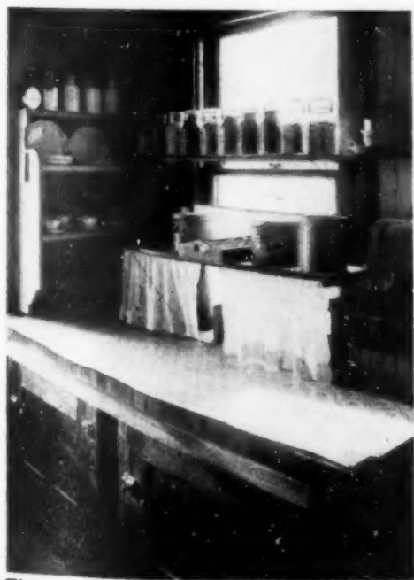
The kitchen table is placed in one corner and made a fixture by building cupboards in the waste space beneath it
