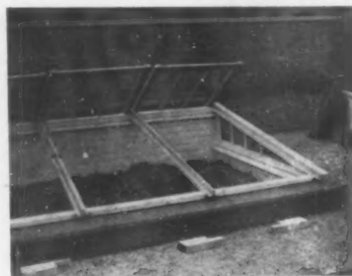
If you build a permanent structure to support the sash you can use it in the early spring as a hotbed and throughout the winter as a coldframe
