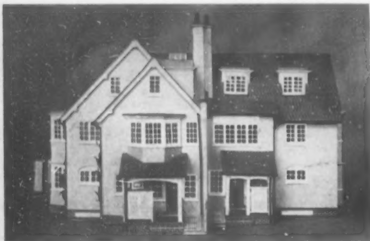
This model was made to show the exact effect of a proposed alteration to an existing building. The change is in the rear bay, which was rebuilt to give a small outdoor sleeping-porch
