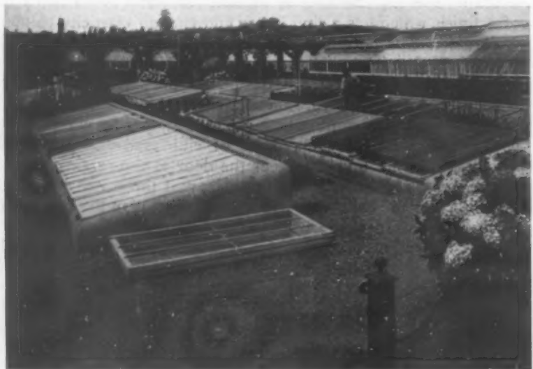
The decay and warping of wooden hotbeds and coldframes is a common fault. Concrete frames will last forever
