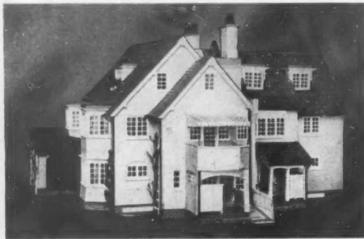
This model was made to show the exact effect of a proposed alteration to an existing building. The change is in the rear bay, which was rebuilt to give a small outdoor sleeping-porch
