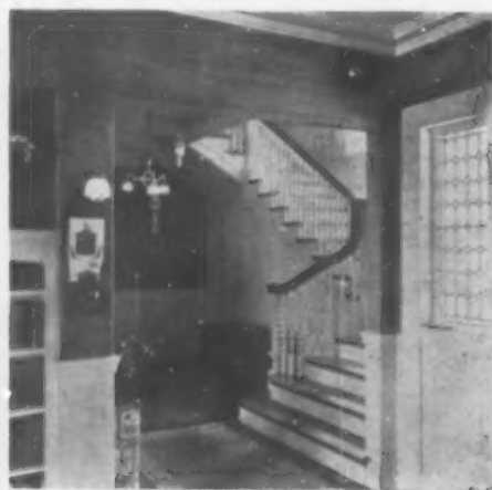
Exterior and Interior Views Showing Blau-Gas Installation
