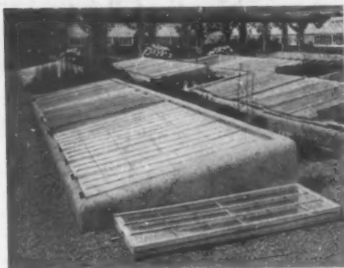
Probably the most economical and serviceable structure is one made of concrete. With some boards, cement and sand, you can make one yourself
