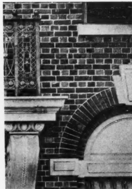
English bond—alternate rows of headers and stretchers, with joints of the latter over one another
