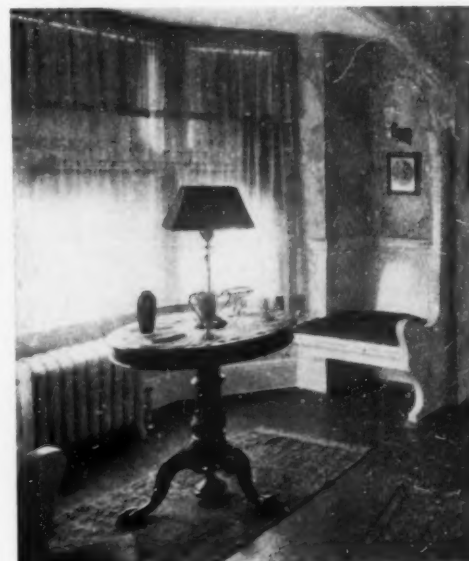
A special radiator enamel is now obtainable so that the iron can be made to match the color of woodwork or wall covering
