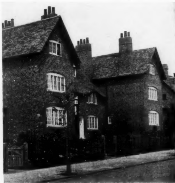
Common running bond in its best form. Every fourth row is one of alternate headers and stretchers to tie the facing brick to the rest of the wall
