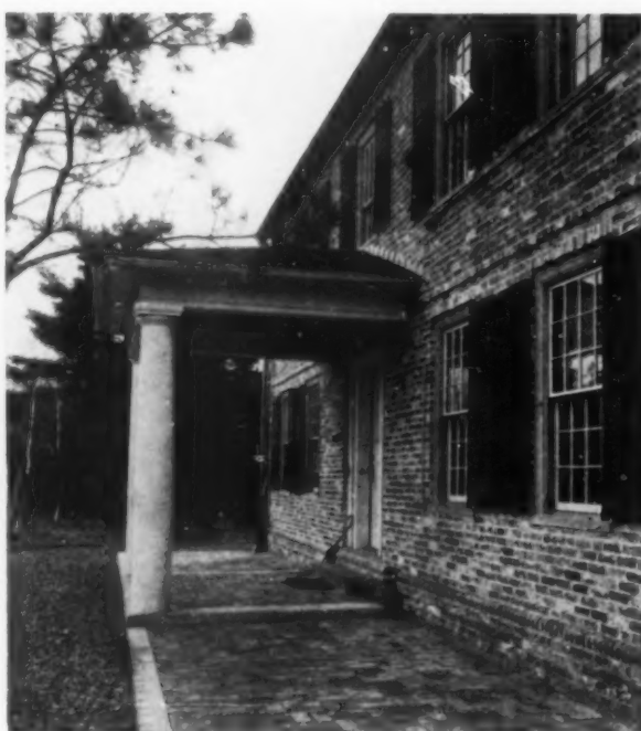
An interesting texture is obtained here with second-hand brick, from which the old mortar has not been fully cleaned. Philip B. Howard, architect
