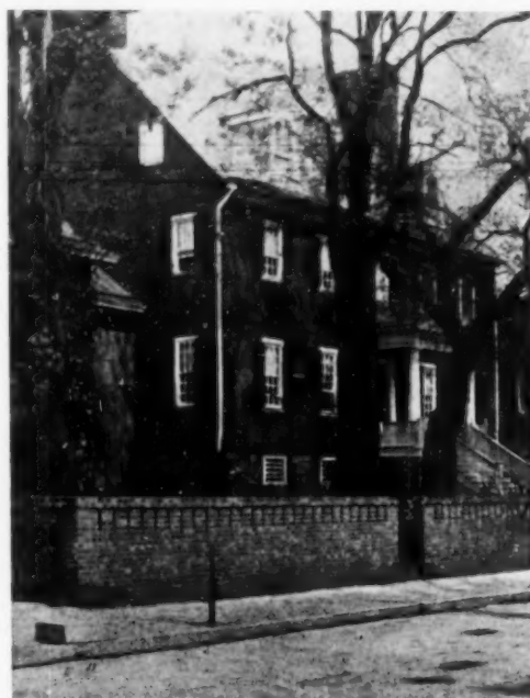
This old Southern mansion and its garden wall are of all-header bond, breaking joints
