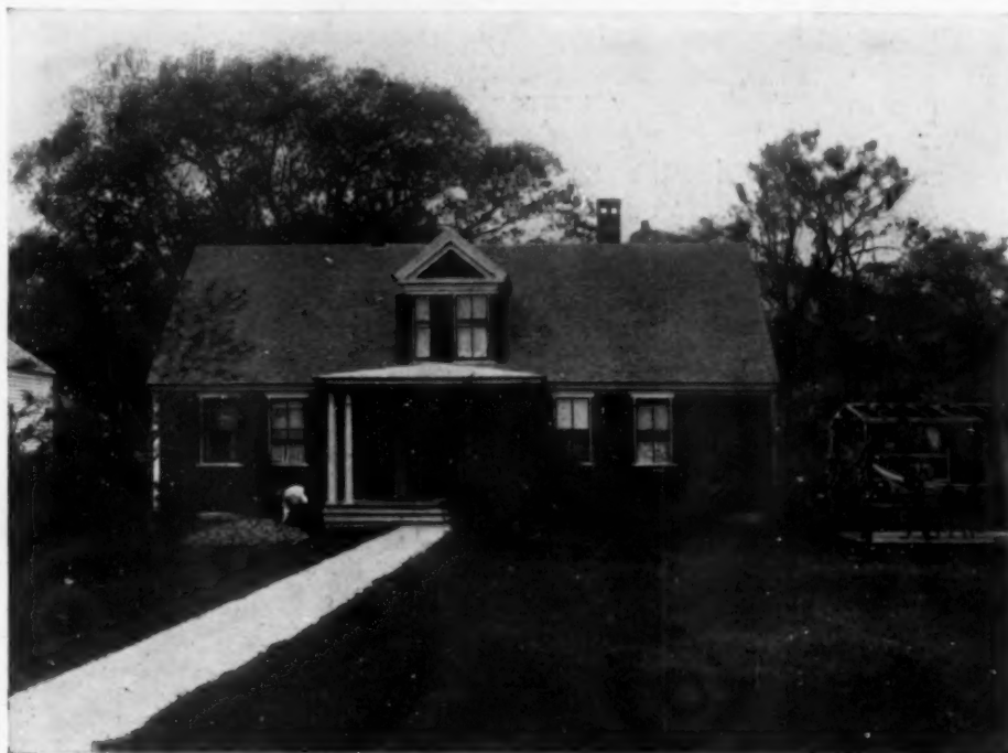
THE OLD HOUSE RESTORED
