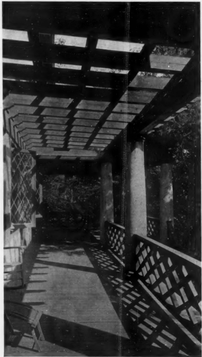
A VERANDA AT THE TENNEY HOUSE
