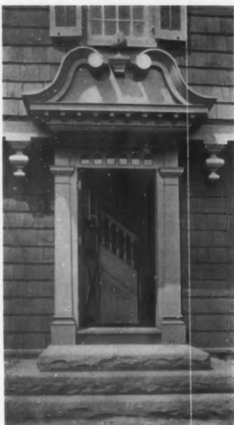
Detail of Entrance
