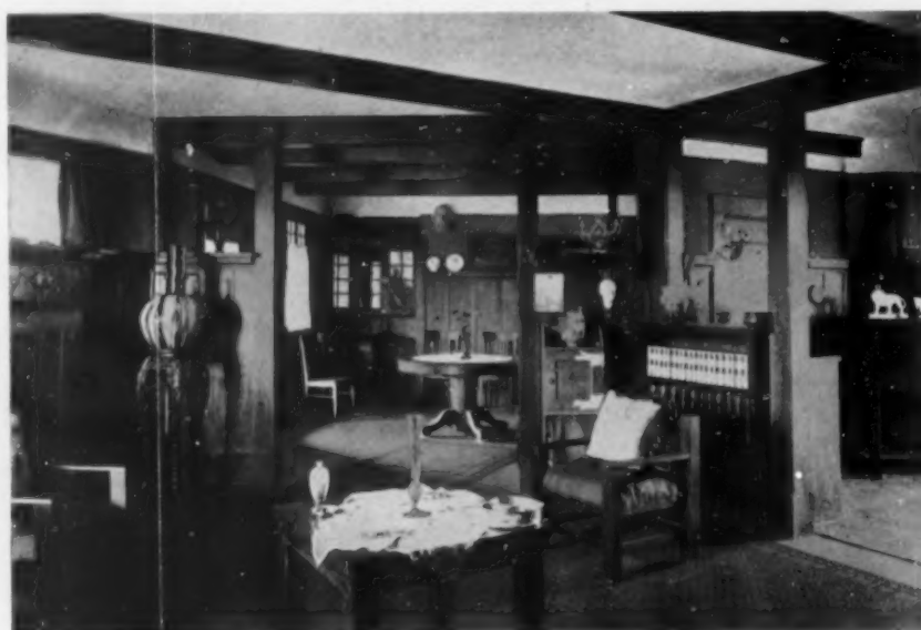
THE DINING-ROOM AND VESTIBULE FROM THE LIVING-ROOM
