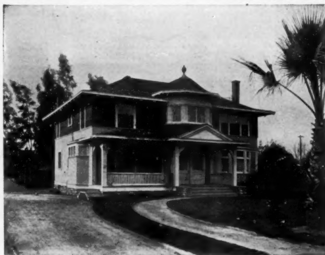
Green & Green, Architects, Los Angeles.
