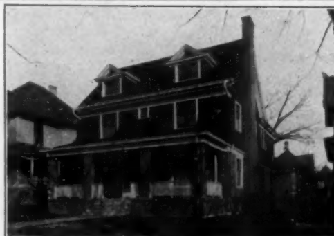
Robinson & Campau, Architects, Grand Rapids.
