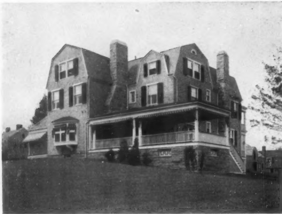
EXTERIOR VIEW OF "HILLSIDE"
