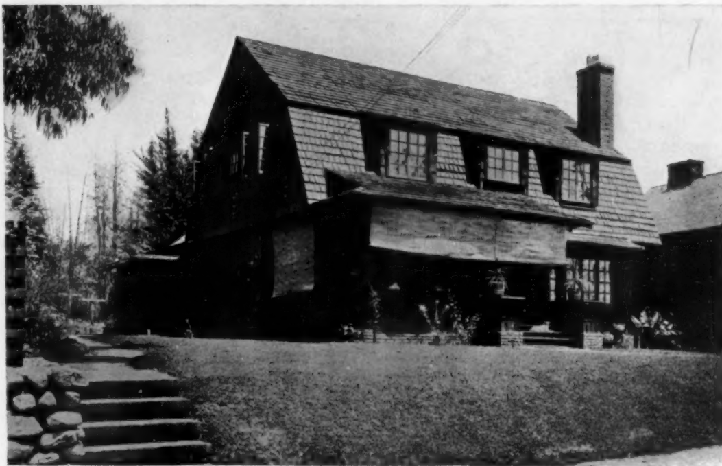
AN EXTERIOR COVERED WITH "SHAKES"
