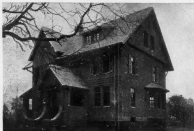
A CONCRETE RESIDENCE, MONTCLAIR, N. J. A. F. NORRIS, Architect.
