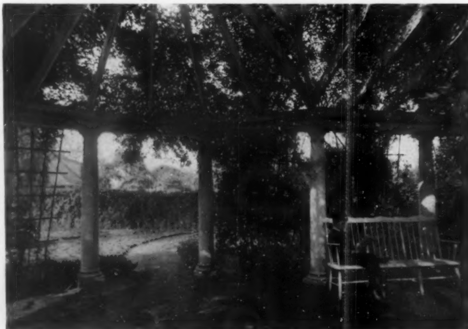
WOOD LANE VIEW FROM THE PERGOLA
