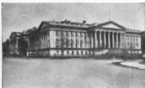
U. S. TREASURY BUILDING, WASHINGTON WE RECONSTRUCTED THE ENTIRE HEATING SYSTEM
