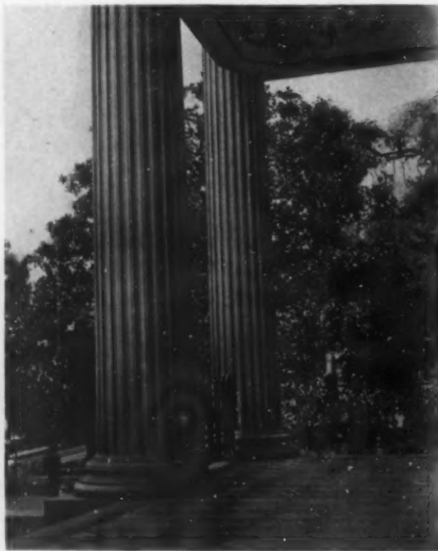
DETAIL—"STANTON HALL" PORCH
