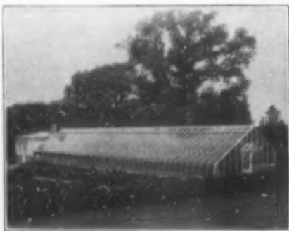
Note the curved eaves—the wonderful lightness of construction.
