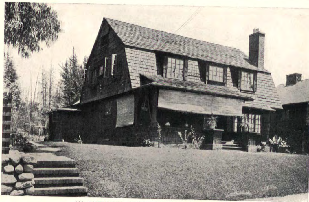
AN EXTERIOR COVERED WITH "SHAKES"
