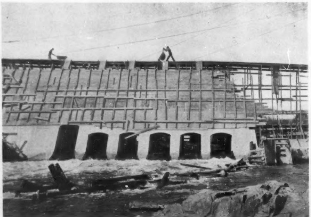
CONCRETE DAM AT SPRAGUE'S FALLS, ME.
