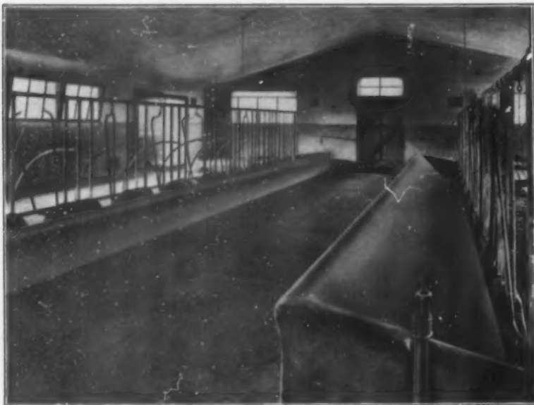
INTERIOR OF CONCRETE COW STABLE Cement Age
