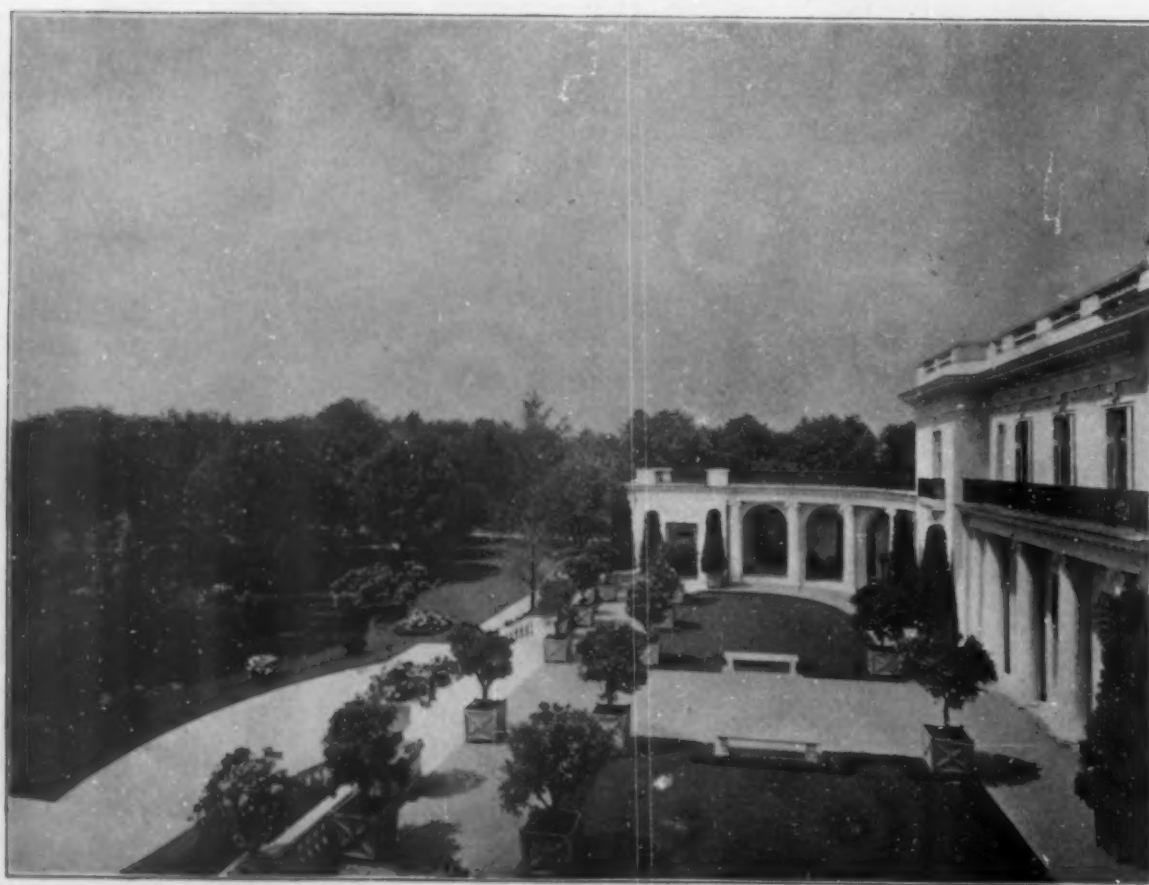
NORWOOD PARK—UPPER VIEW OF THE TERRACE
