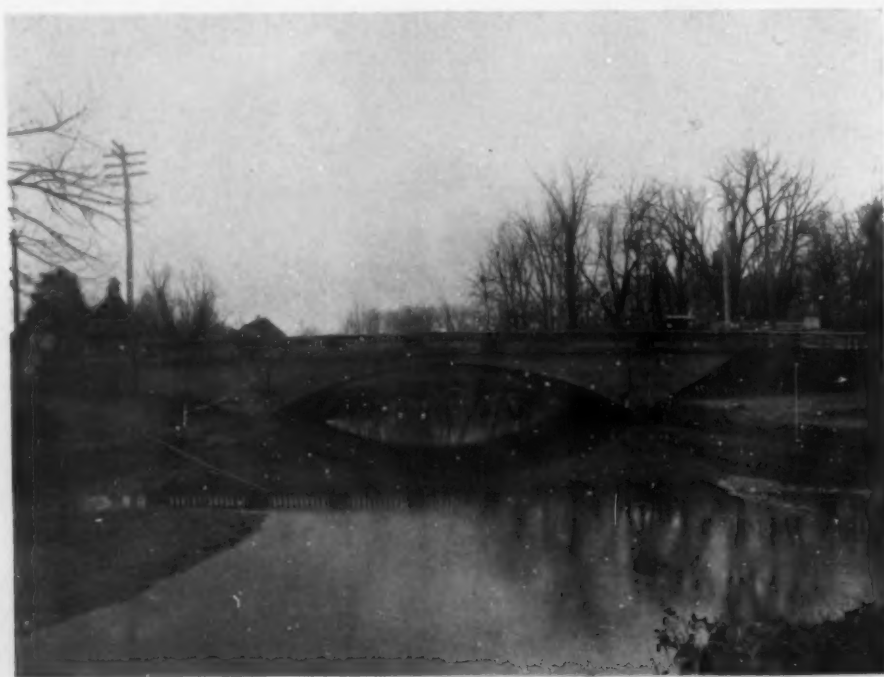
CONCRETE BRIDGE OVER POQUESSING CREEK, PHILADELPHIA. THIS BRIDGE HAS A SPAN 71 FEET WIDE, WITH A RISE OF 9½ FEET Cement Age
