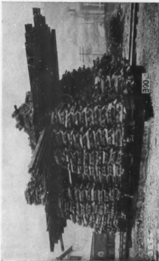
Test load of 300 tons on five concrete piles, Westinghouse Works, Pittsburgh. This is the heaviest test load ever placed on piles of any kind, and was carried by the piles without difficulty
