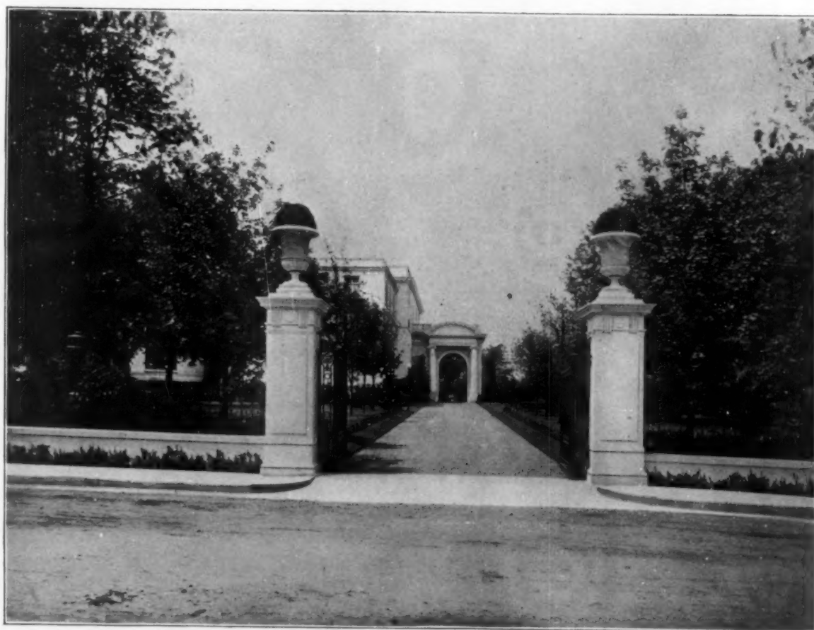
NORWOOD PARK—THE ENTRANCE GATES
