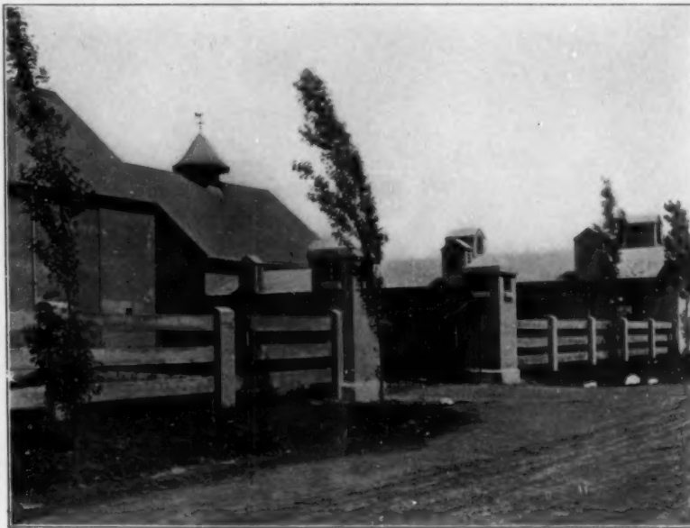
CONCRETE WORK ON THE FARM
