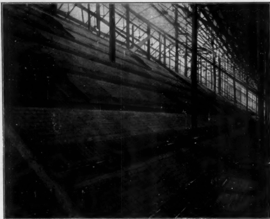
WIRE CLOTH IN PLACE READY FOR THE CONCRETE Interior of Government Coal Pockets, Bradford, R. I. Clinton Wire Cloth Co.
