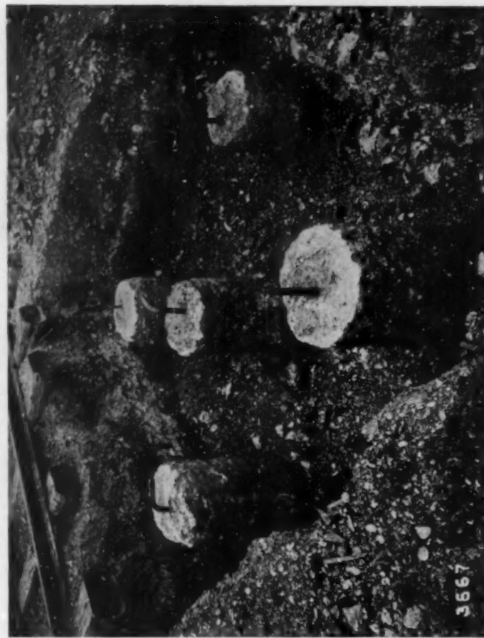
The five piles which bore the test shown above. This photograph shows the piles ready for the concrete "cap," upon which the load rests
