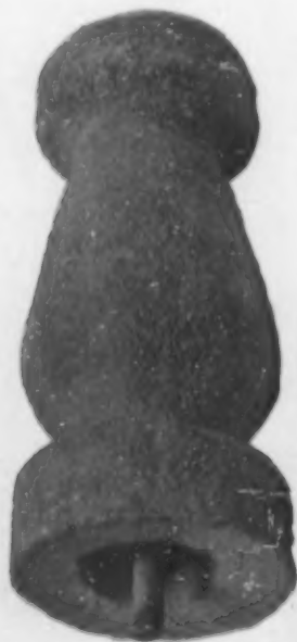
CONCRETE BALUSTER IN A PHILADELPHIA BRIDGE, SHOWING ROUGHENED SURFACE, SOMEWHAT LIKE PEBBLE DASHING
