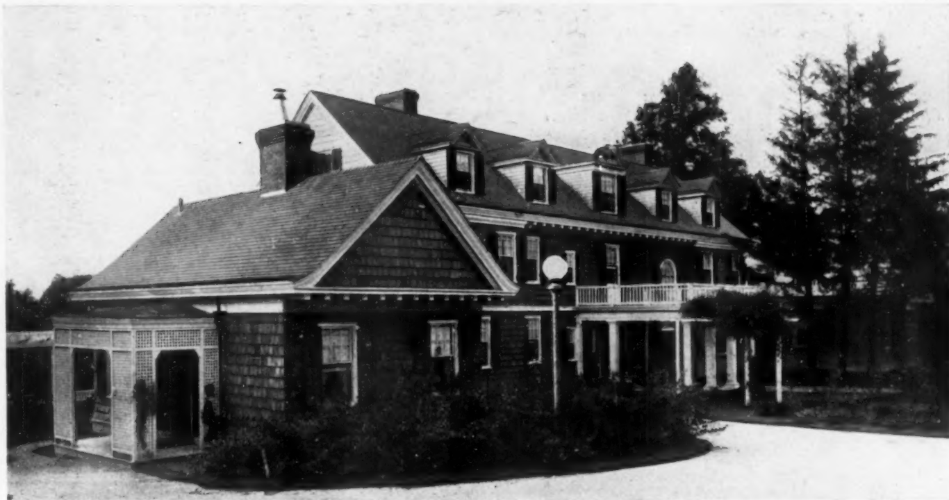
VIEW FROM THE NORTHWEST
