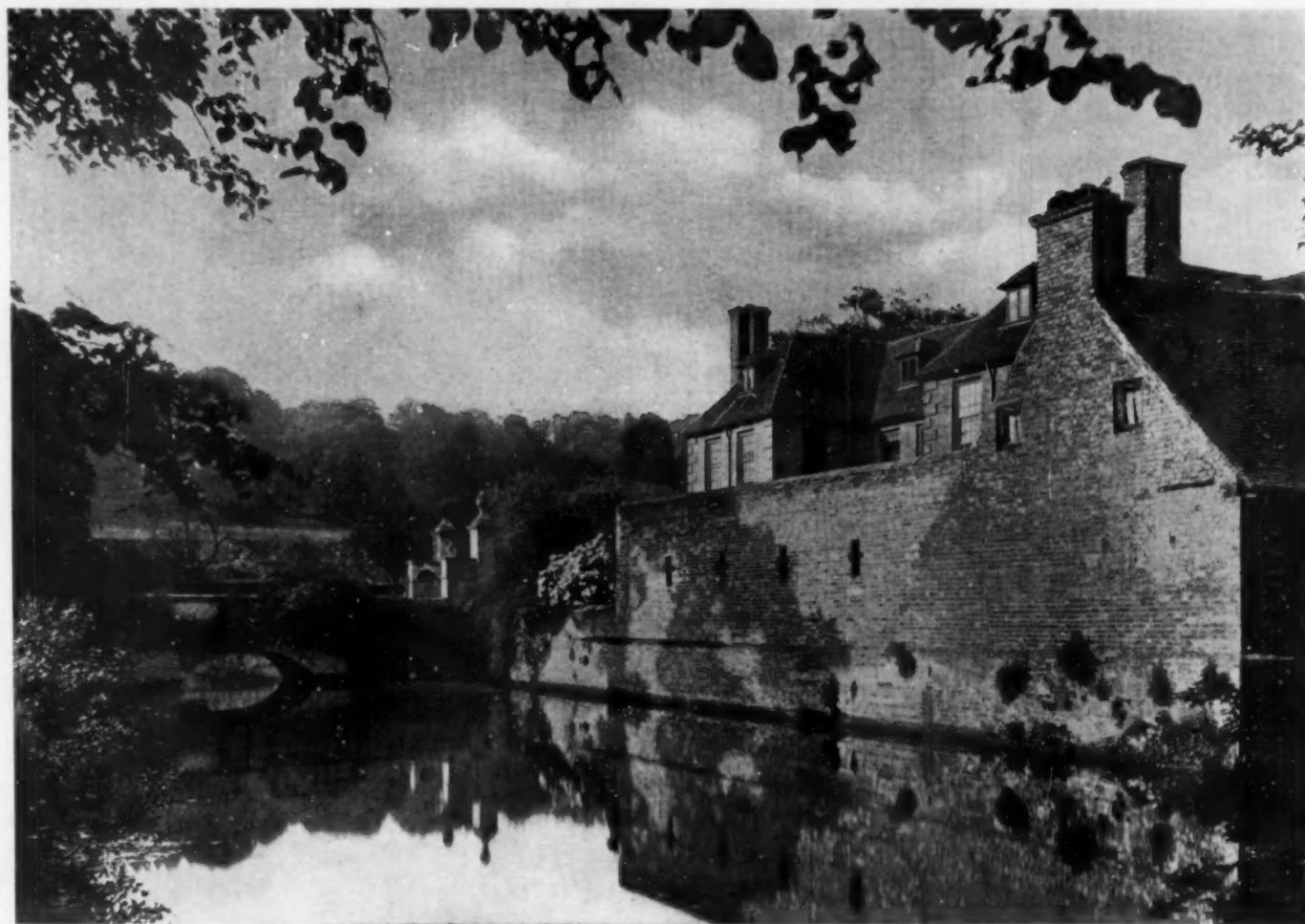
GROOMBRIDGE PLACE, KENT. THE WEST BRIDGE
