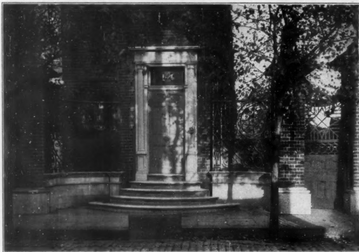
DOORWAY OF EDMONDSON HOUSE
