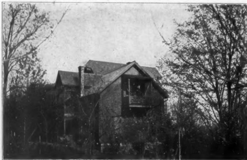
A SECOND STOREY BALCONY
