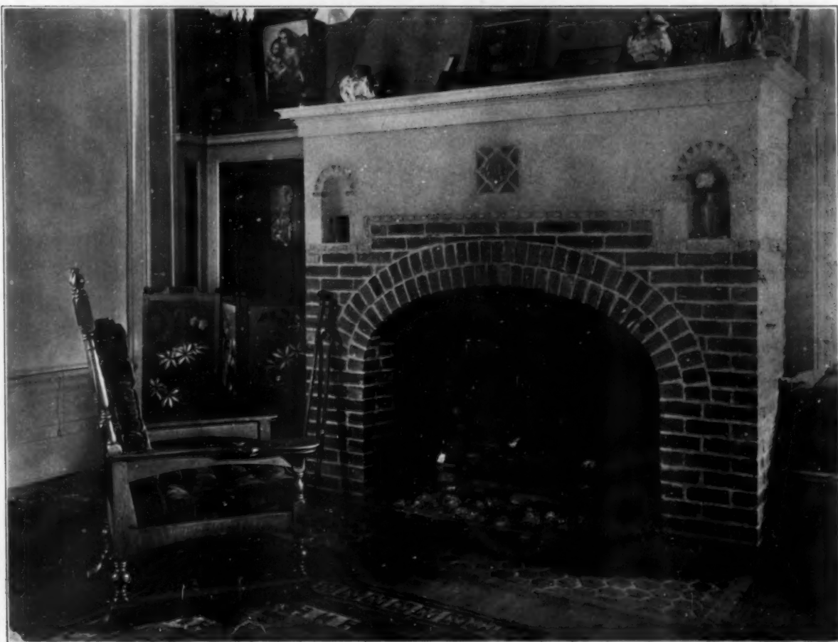
ROUGH BRICK FIREPLACE WITH TILE INLAYS IN PLASTER
