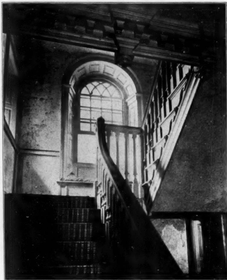
THE STAIR LANDING
