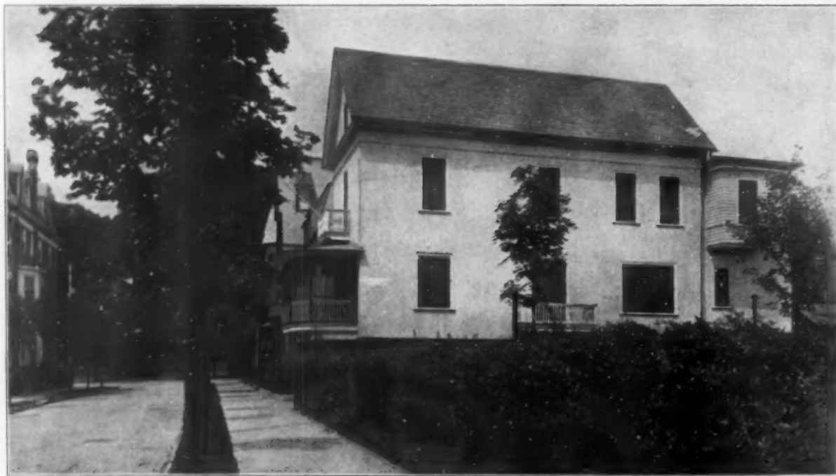
THE SOUTH WALL
