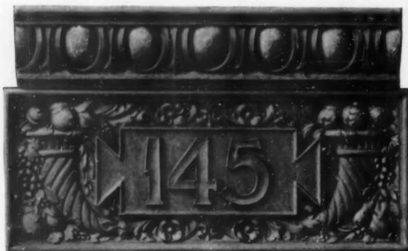
A FRIEZE PANEL FOR THE 145TH STREET STATION Executed by the Atlantic Terra-Cotta Co.
