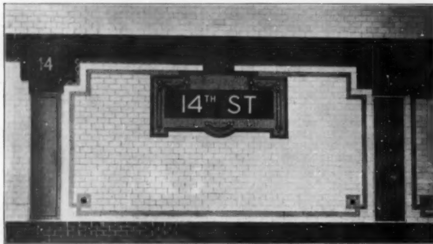
THE EAST WALL AT THE 14TH STREET STATION
