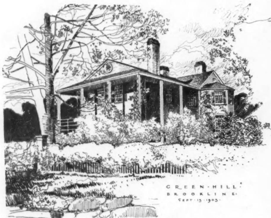
THE PILLARED VERANDA
