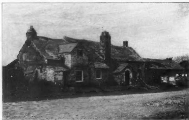
HOUSES ROOFED WITH STONE
