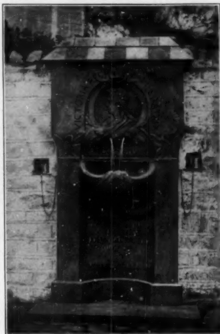
A STREET FOUNTAIN IN CLOVELLY By Countess Feodora Gleichen
