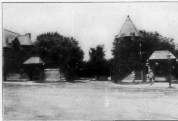
ENTRANCE TO PORTLAND PLACE Theo. C. Link, Architect
