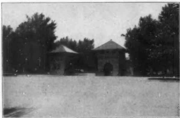
ENTRANCE TO WESTMORLAND PLACE Eames & Young, Architects
