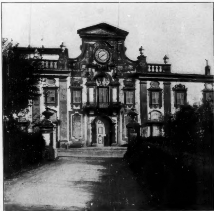
THE ENTRANCE FROM THE PUBLIC ROAD
