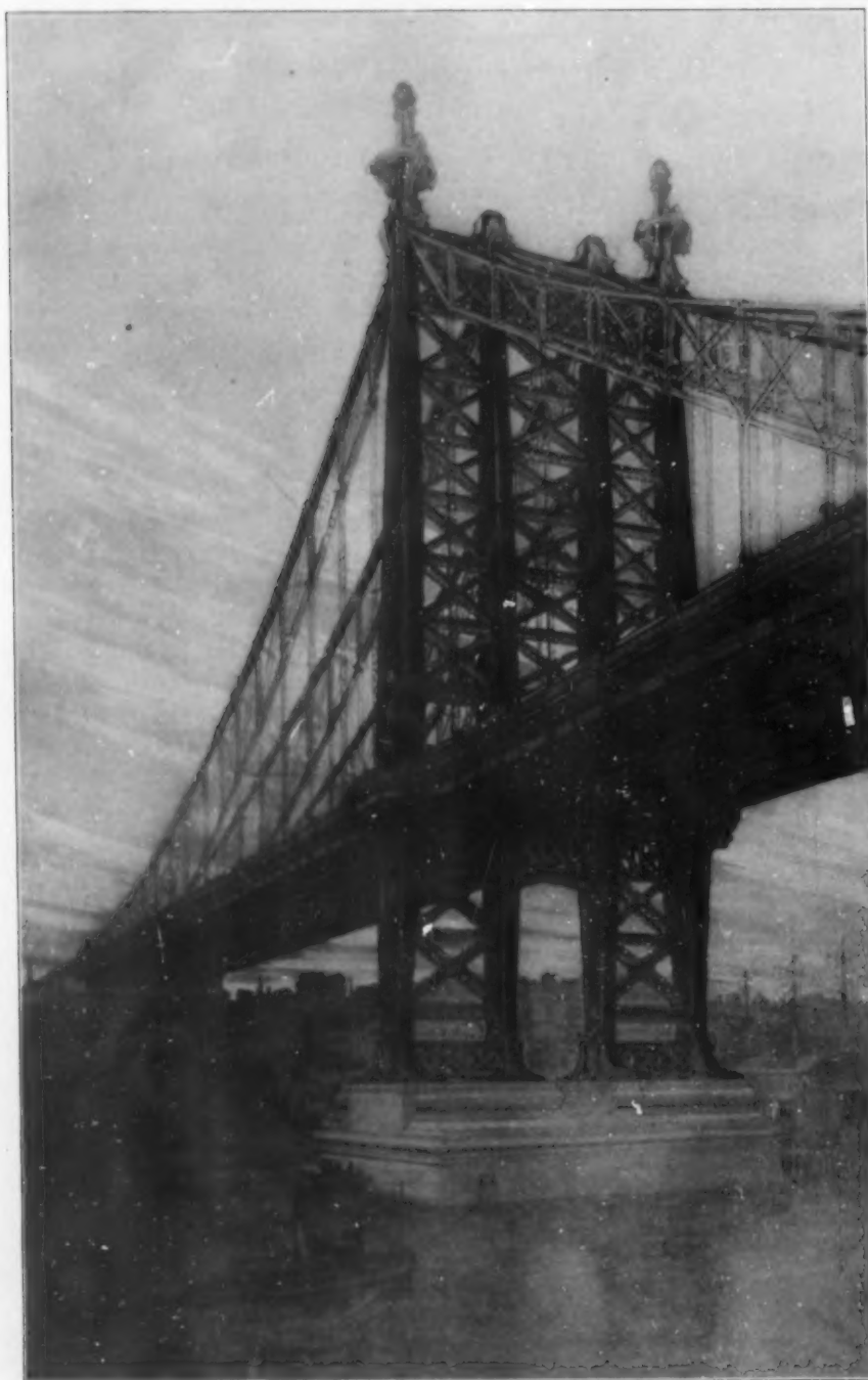
A PIER OF THE MANHATTAN BRIDGE
