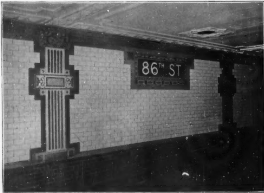
A TYPICAL UP-TOWN STATION
