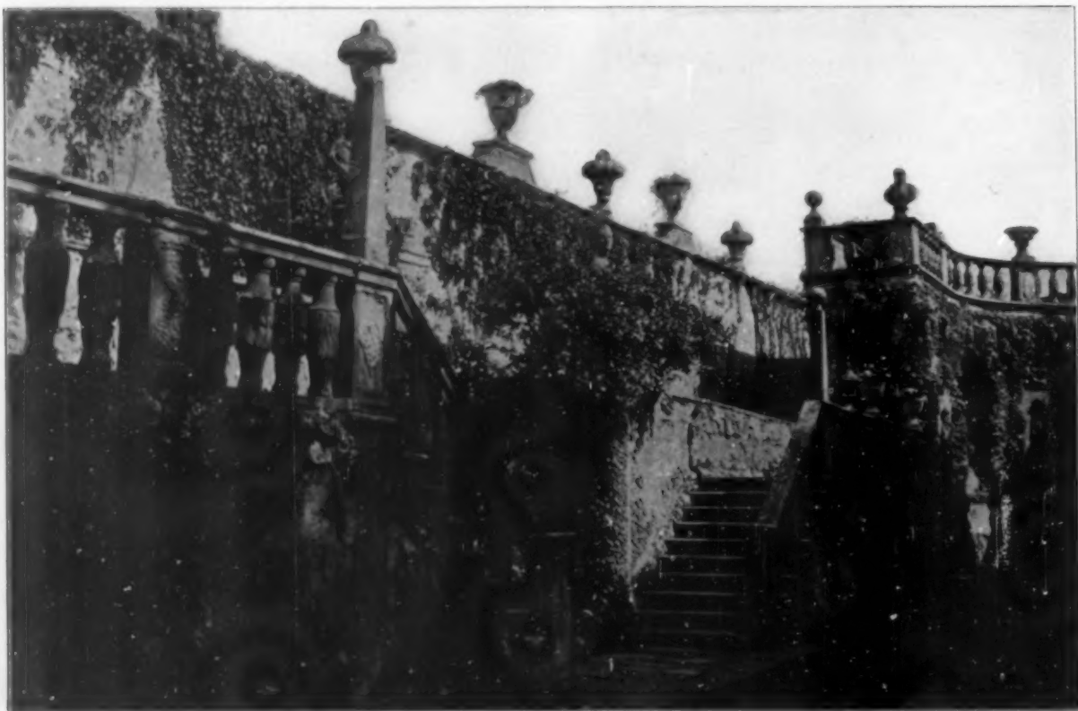
THE RETAINING WALL OF THE OLD GARDEN COURT Showing the applied rock work of the Eighteenth Century
