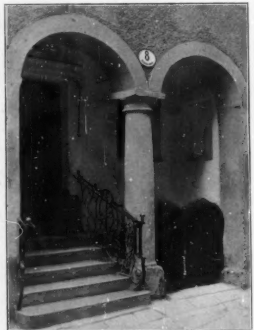
A TYPICAL HOUSE ENTRANCE
