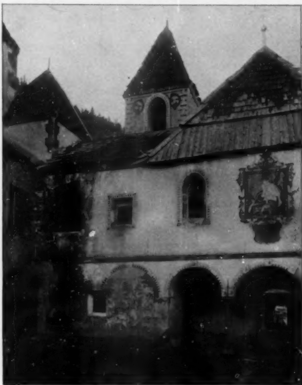
COURTYARD OF FISCHBURG
