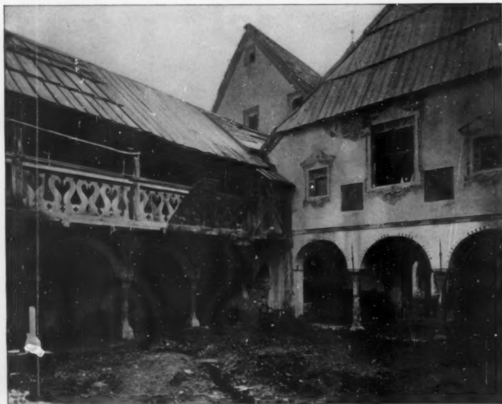
COURTYARD OF FISCHBURG
