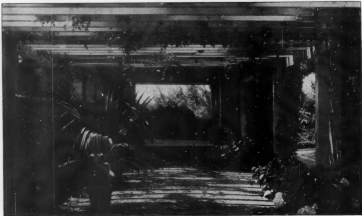
THE PERGOLA FROM THE NORTH END
