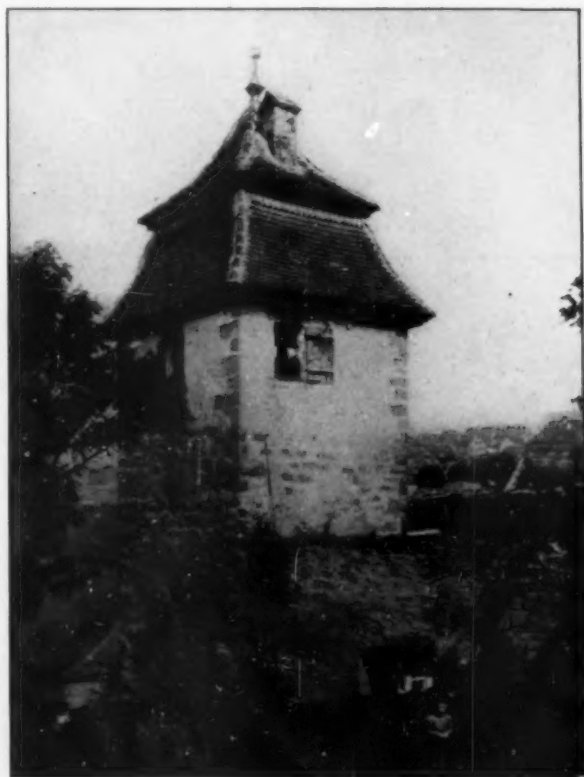
THE KOBELZELLERTHOR TOWER
