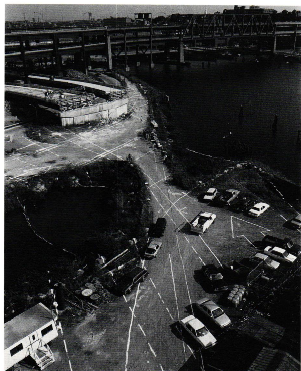
Kennedy and Violich Architecture with Linda Pollak and Matthew VanderBorgh, Drawing on Site , installation overview, Charlestown, 1990.
