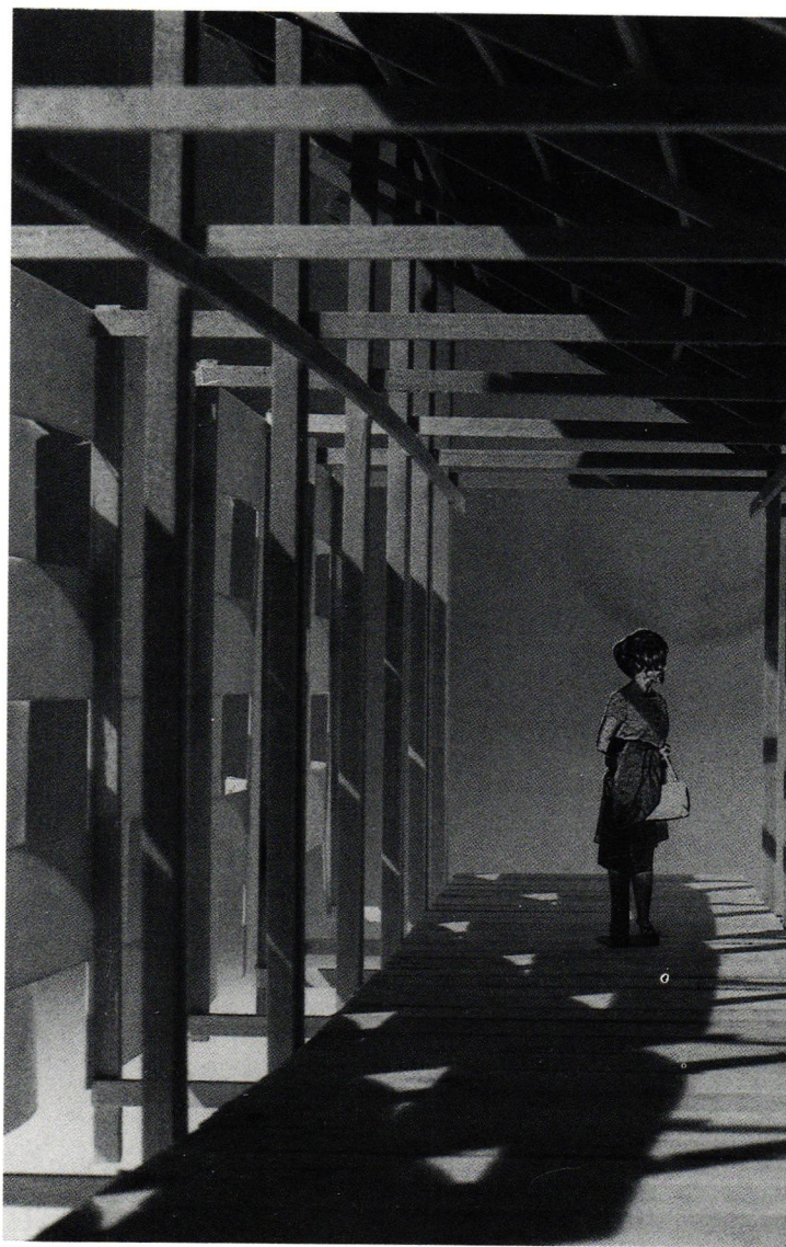
Commuter Bridge, interior view at junction with Bent no. 62.
