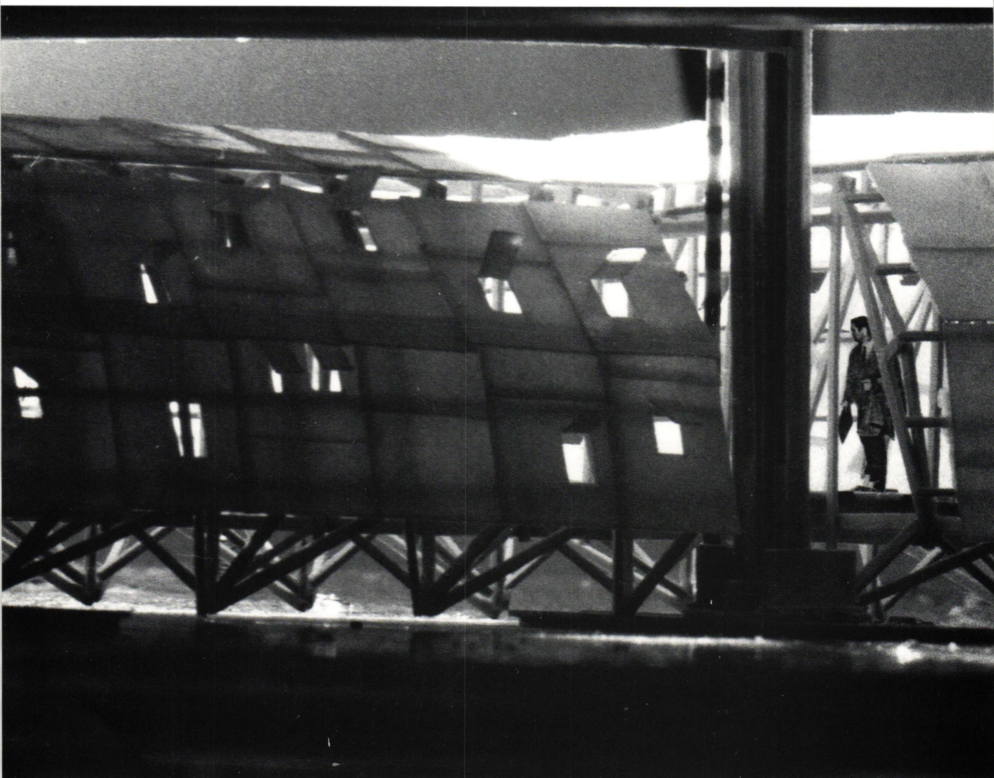
Listening Bridge, view of skin at intersection with Bent no. 43.
