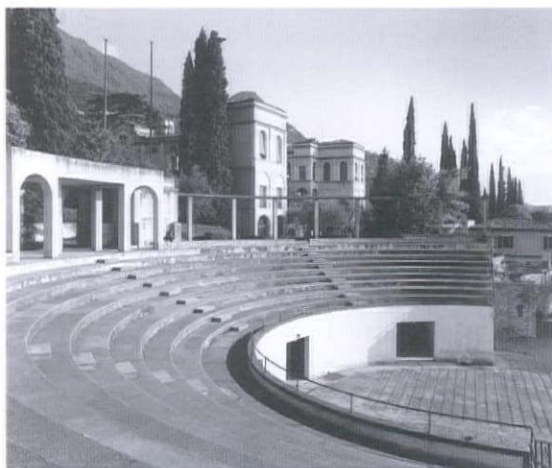
21. The Theater, under construction by 1934 and completed in 1953.
