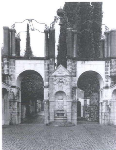
25. The entry gate
