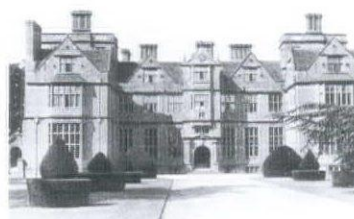
Figure 21. Condover Hall, by Walter Hancock (mason), Saalop, Shropshire, (1598); Mullioned window and gable at left side wing.
