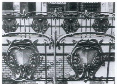
Figure 24. A detail view of a railing at a Metro Station in Paris, by Hector Guimard, circa 1900.
