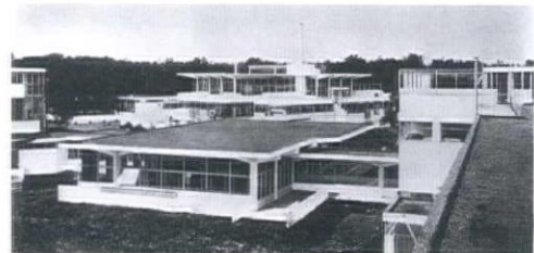
Figure 19. View of the recently completed Zonnastraal Sanatorium by B. Bijvoet and J. Duiker, Utrecht, Holland, 1928; an example of the high point of "sachlich" technocracy.
