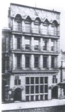
Figure 2. Birmingham offices for the Eagle Insurance Company by Lethaby. Note the rhythmic variations of the fenestration, responding to the internal layout of spaces and their function. The entrance level served as a large customer transactions hall, whilst the upper levels housed individual office rooms.
