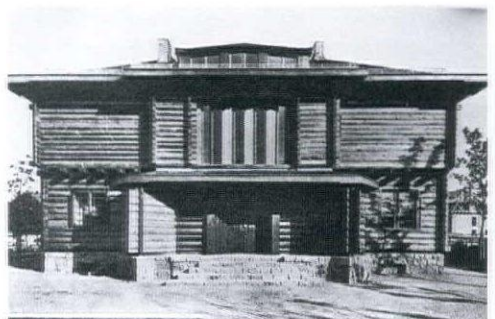
Figure 4. The highly handcrafted Sommerfeld House, Berlin-Dahlem, 1921, by Walter Gropius and Adolf Meyer.
