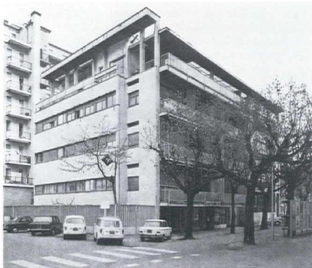
37. Giuliani Frigerio Apartment Block, corner view from which a planar reading is revealed.
