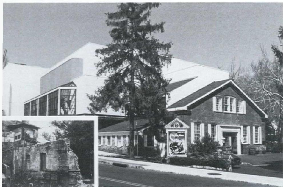
Inset page: Workers restore the ceiling of Strand Theatre. The Paper Mill Playhouse (inset) bounced back after being destroyed by fire in 1980 (inset).
