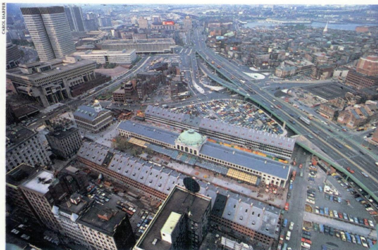
Bounded by the Southeast Expressway (top), Government Center (left), and the financial district (lower right), Boston's recently restored Faneuil Hall Marketplace is one of the country's most successful shopping centers.
