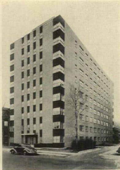
Aluminum Windows in Abbottsford Apartment Building, Milwaukee, Wisconsin. Buecking & Jahn, Architects.
