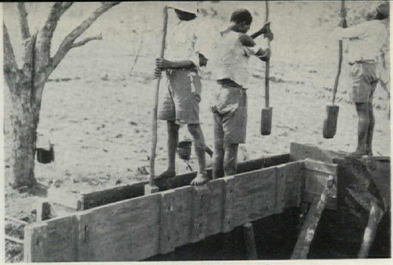
Tamping Pise-de-terre walls.
