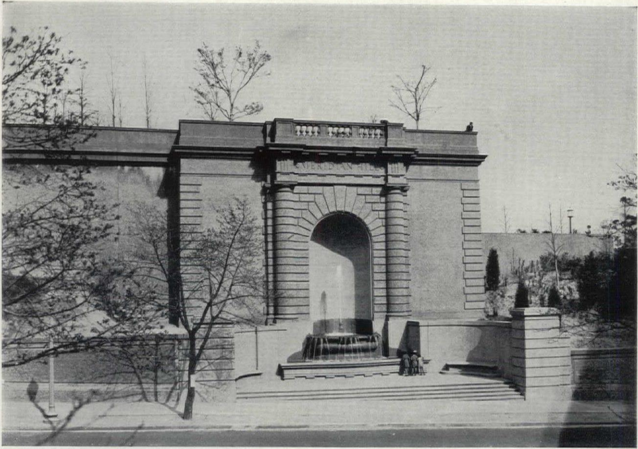
PYLON AT MERIDIAN PARK
