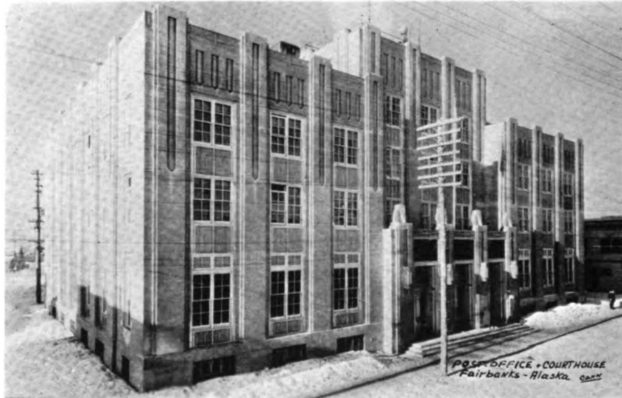
UNITED STATES POST OFFICE AND COURT HOUSE, FAIRBANKS, ALASKA Office of Supervising Architect, Architect
