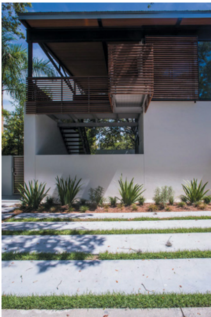
Exterior terrace showing one of two exterior stairs that create an indoor-outdoor circulation loop.
