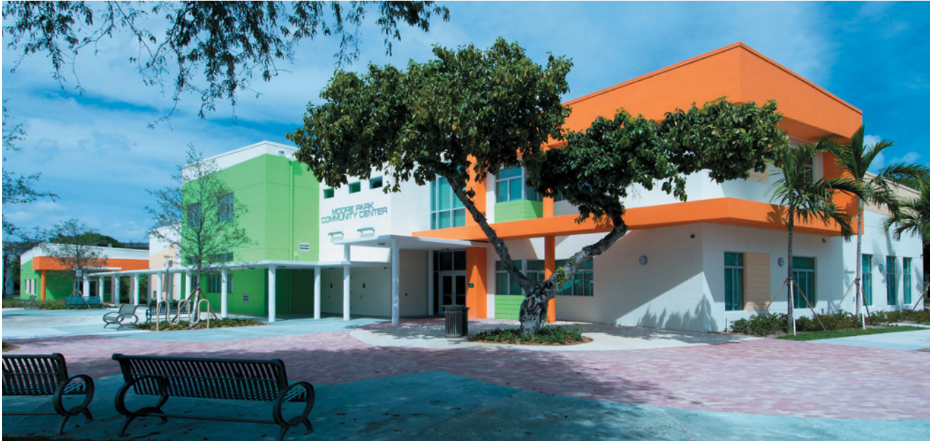
The main entrance to the community center. Sited in a vibrant Miami neighborhood, the center is an expression of local tradition. All photos by Chuck Wilkins.
