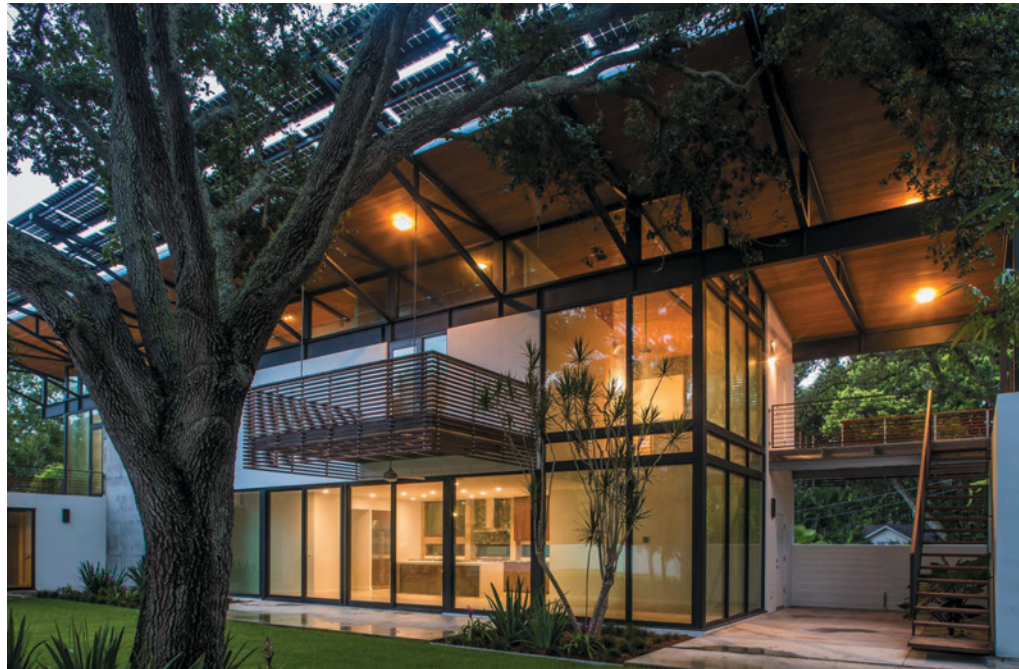
North elevation facing the courtyard. All photos by Bill Speer.
