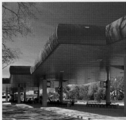
VOTRAN designs transformed a standard requirement for protection from the elements into a sculptural, provocative feature of the facility.
