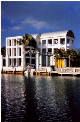
The front elevation turns its back on the street in favor of large glass areas and views to the canal. Photograph: Carlos Domenech
