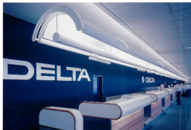
Reclining fixtures provide a pleasant glow and comfortable task lighting for ticket agents.
