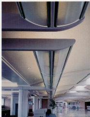
In each concourse, custom indirect light fixtures bracketed off the columns provide ambient lighting to supplement daylight from the windows and continuous skylights.
