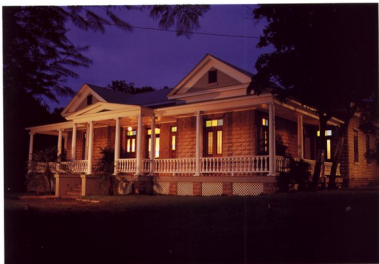
Frost facade. The interest of the divided facade is accentuated by night-time lighting. The initial phase of the project included restoring structural integrity, replacing deteriorated elements, and harmoniously integrating new modern electrical and mechanical systems. Photograph: Agnieszka Gus Postel, Ph.D.
