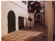
Courtyard, looking toward east gate, where passage is marked by one of several arched masonry stairs. Photograph: Ryce Stallings
