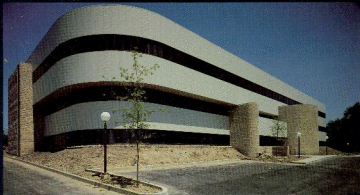
Four Parker Plaza, Pittsburgh, Pennsylvania. Architect: Williams-Tierlinck-Wheathead. General Contractor: Melton/Sloan Co.
