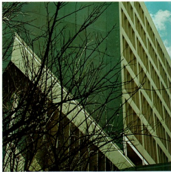
Above: Coral Gables House, Coral Gables; Architect: Bureau, Bernello, Kushi & Voss, Inc.; Miami; Bottom: State Regional Service Center, Miami; Architect: Russell, Martinez & Holt, Miami; Photo by Dan Foster
