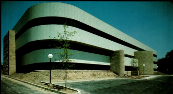
Four Foster Plaza, Pittsburgh, Pennsylvania Architect: Williams - Trebitcock - Whitehead General Contractor: Mellon-Stuart Co.
