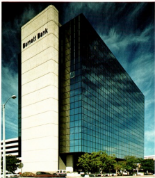
Above: City of Miami Police Headquarters, Miami; Architect: Pinzaut Architects and Rudenno Barred-ly Atlanta, Miami; Below: Douglas Center Office Building, Coral Gables; Architect: Nicholas Fuller-ton & Associates, Coral Gables; Photo by Steven Bruck
