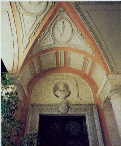
Top: Doorway detail, Victoria, Miami.
