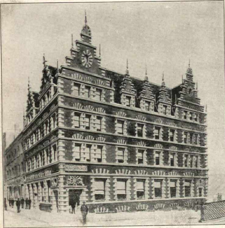
NEW CHICAGO OFFICE BUILDING, IN COURSE OF ERECTION.
