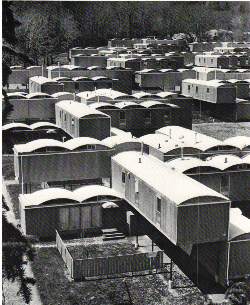
Oriental Masonic Gardens, New Haven, Connecticut, 1971, a "plug-in," movable housing development by Paul Rudolph, using units fabricated in Baltimore, Maryland and trucked to the site
