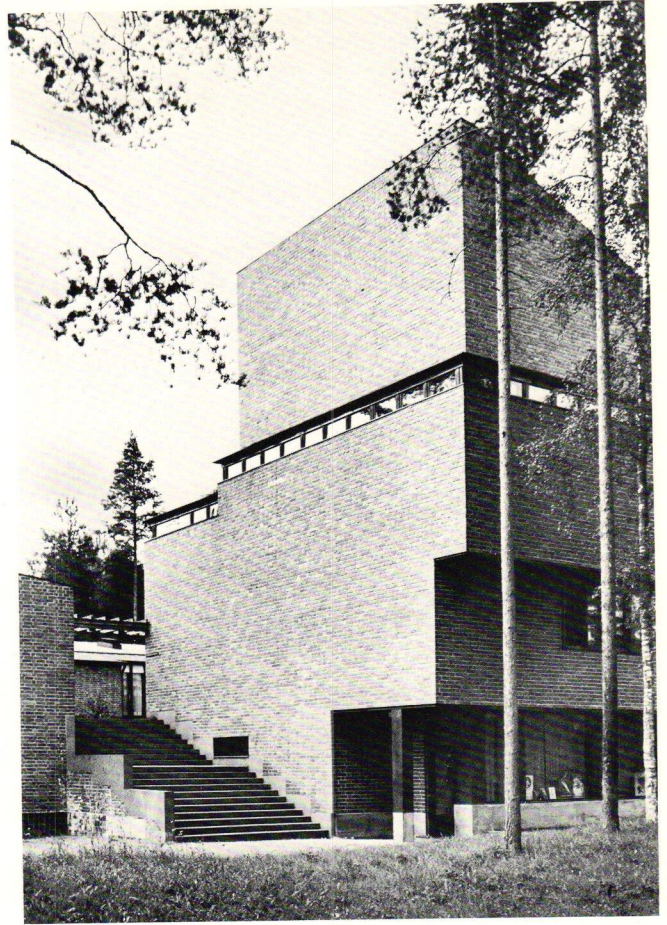
Aalto , Civic Center, Säynätsalo, 1951, closed brick envelopes, Aalto's strong individualism, the 50s
